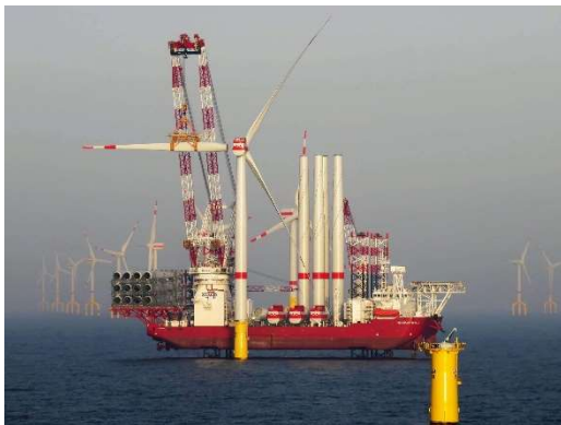
Wind turbine installation vessel (WTIV)
