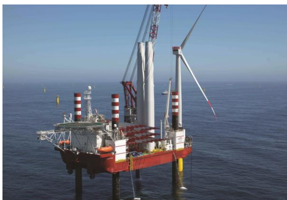
Self-elevating platform (Ship : Wind Zaratan)
